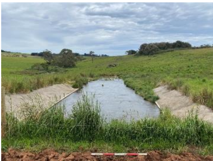
Plate 9: General area shot showing culvert on dissected plain landform (facing south).
