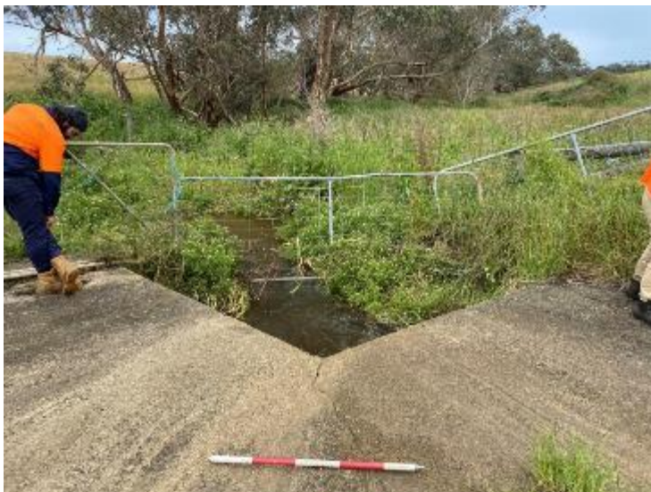
Plate 8: General area shot showing culvert on dissected plain landform (facing south).
